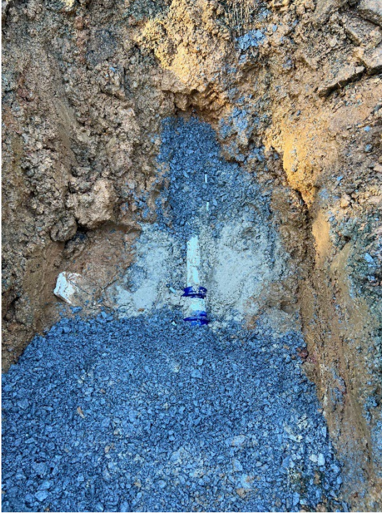
Main Line Repair – 29 Labor Hours | Excavator, Service Trucks, Ditch Witch, Dump Truck
