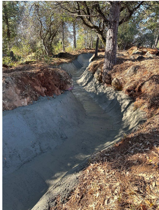
Canal Lining – 42 Labor Hours | Excavator, Service Trucks
