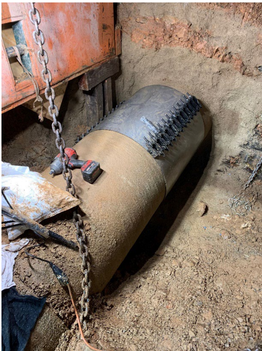
Raw Water Conduit Repair – 116 Labor Hours | Excavators, Dump Trucks, Traffic Control, Service/Utility Trucks, Locating, Emergency Contractor Work
