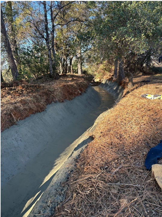
Canal Lining – 42 Labor Hours | Excavator, Service Trucks
