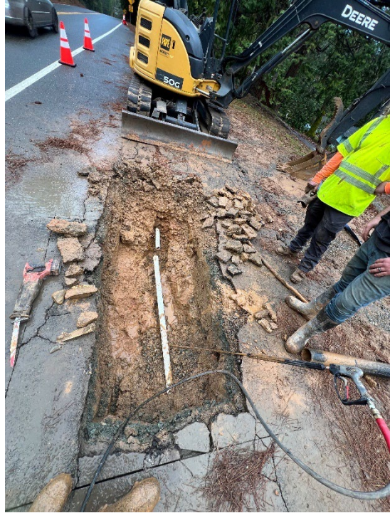
Main Line Repair – 29 Labor Hours | Excavator, Service Trucks, Ditch Witch, Dump Truck
