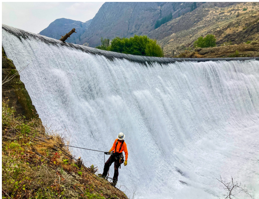
Figure 2. Enloe Dam Dewatered Inspection, Geologic Reconnaissance, Oroville, Washington, USA
