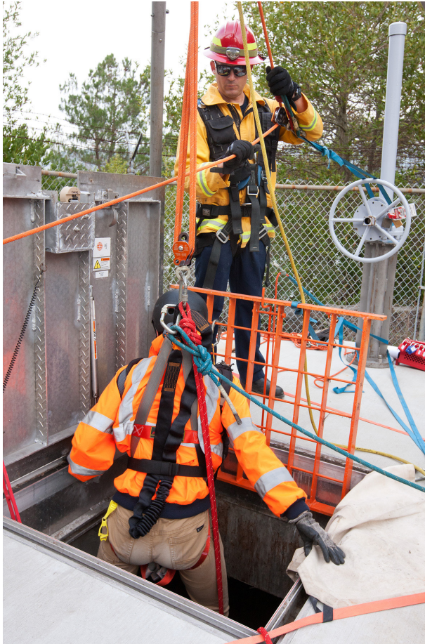
Figure 6. San Pablo Tunnel Inspection; Capstone lowering inspector down into East Shaft
